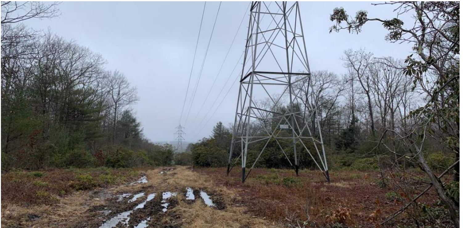
Photo #4: View of existing Structure 401, ORW BVW PE-W6A and intermittent stream PE-SC6A (Str 402 in background). B-402 is proposed approximately 18 feet northwest of the existing structure. Temporary construction matting in ORW BVW PE-W6A is required in order to access B-402 located in the 100-ft Buffer Zone. The access to the boring will also span PE-SC6A. Facing northwest.
