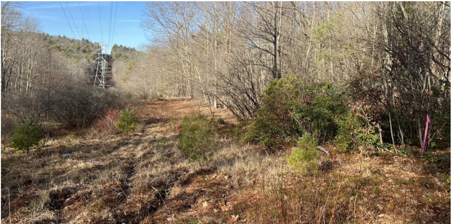
Photo #6: View of BVW PE-W2 (Str 421 in background). Temporary construction matting in ORW BVWs including PE-W2 is required in order to access B-421 located in upland. Facing northwest.
