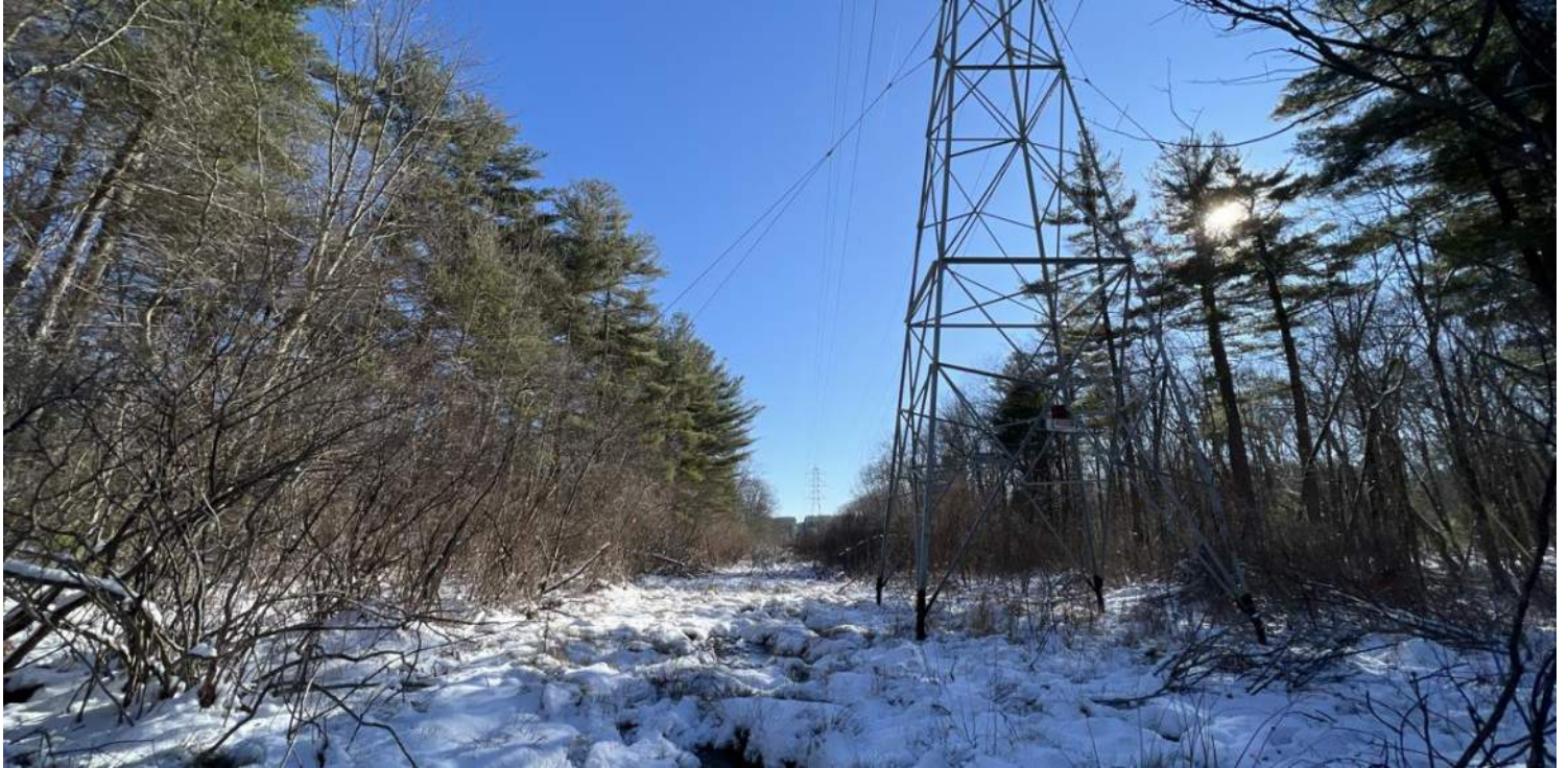
Photo #1: View of existing Structure 377 located within ORW BVW PE-W20. B-377 is proposed approximately 18 feet southeast of the existing structure. Temporary construction matting in BVW is required in order to access and create a work envelope for the work. The access to the boring will also span intermitted stream PE-S6. Facing southeast.
